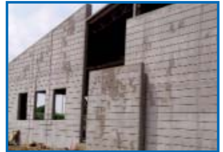
T-Mobile Call Center, another CD 2 project built in record time.
